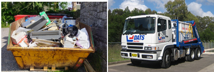
Photograph 2.1 Example of co-mingled construction waste and a typical skip bin truck
